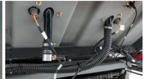
Tank pressure sensors.
